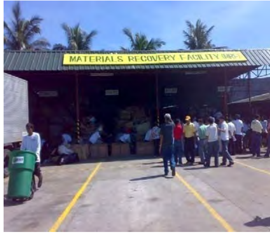
Figure 2. Material Recovery Facility
