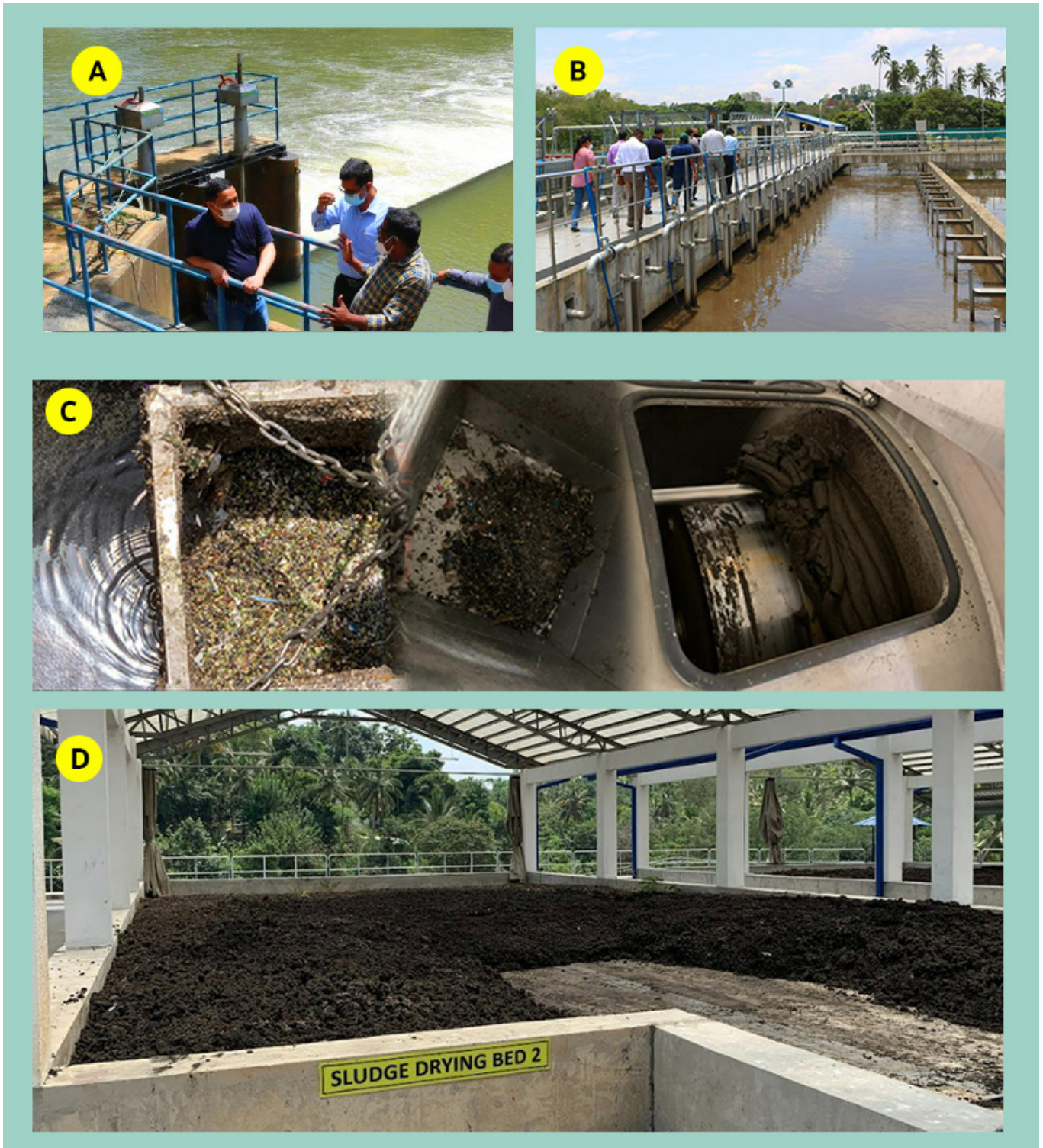
Figure 11. Field photos: a) Water treatment plant intake, b) wastewater treatment plant, wastewater treatment plant strainers retain sludge with visible meso- and large-sized microplastics, and d) sludge drying facility
