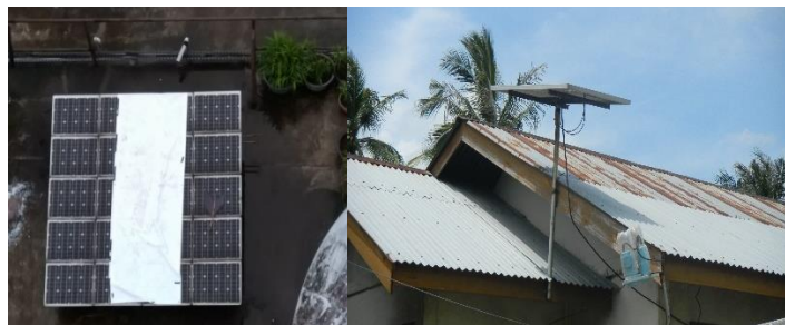
Figure 22. Rooftop solar PV in commercial building
