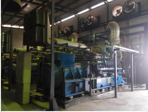
Landfill gas recovery
