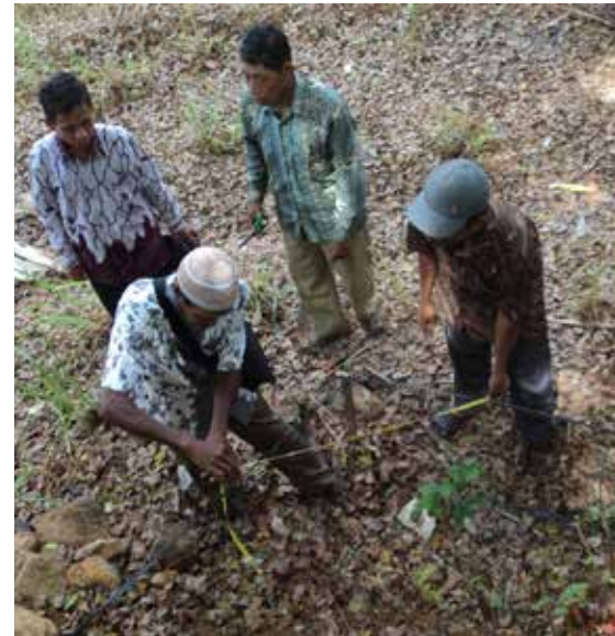
Figure 9. 3-4-5 method to make a square corner
