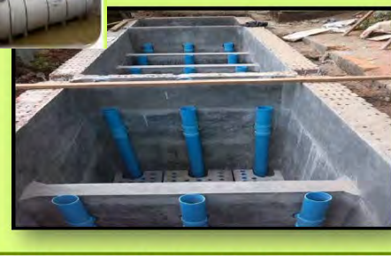
(BORDA) Decentralization Wastewater Treatment System (7m 3 /day) at B.E.H.S (1) Tamwe, Yangon
