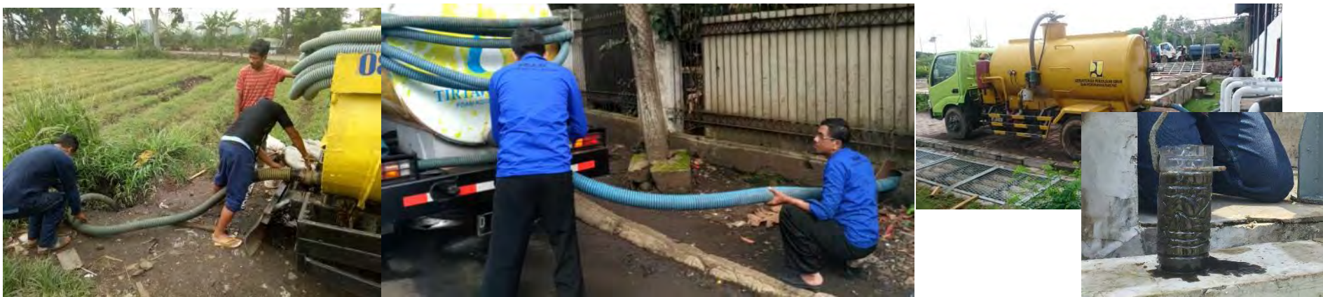
Fig. 1. Discharge of collected septage at “dumping points” in Bandung; and effluent from septage treatment plant in Denpasar, Indonesia (Source: Author)
