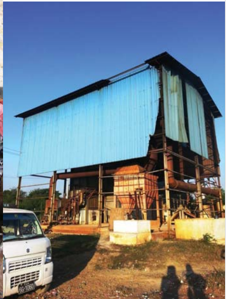
In corner of land fill site is an incinerator for burning clinical wastes (such as syringes)- Chinese technology, poor design, no flue gas treatment
