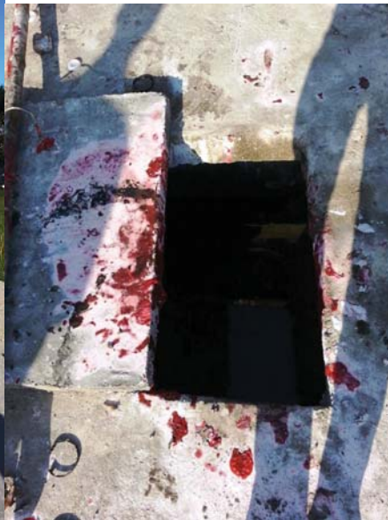
At the Htein Bin cemetery complex, hazardous waste from industries (managed by YCDC) is contained in under ground brick-walled chambers
