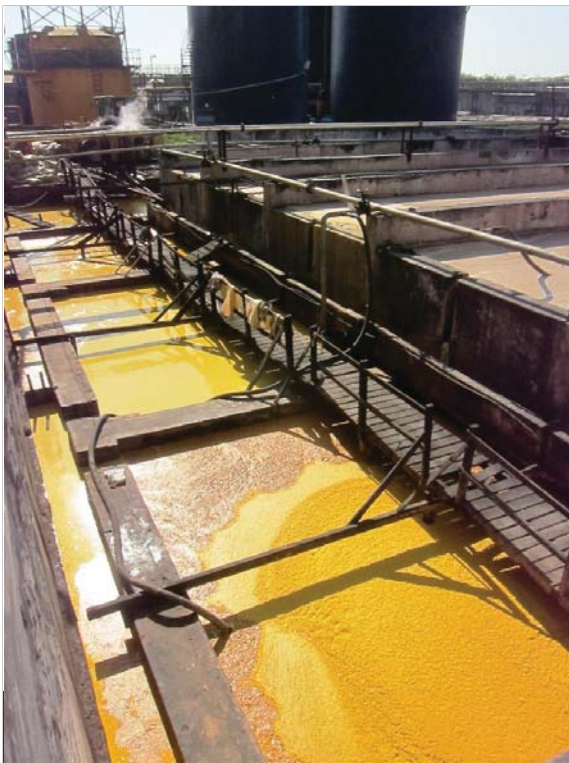
Waste water has high suspended solids; the water is aerobically and anaerobically treated; methane is captured and used as fuel
