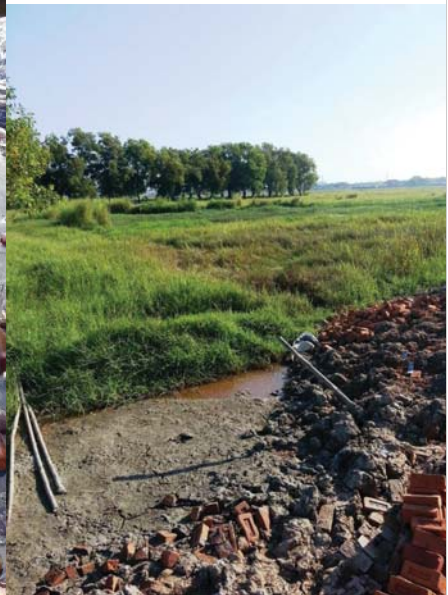
One brick-thick pit; leachates can be seen in adjoining fields
