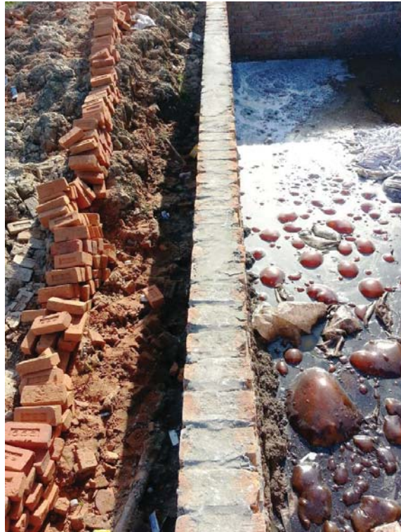
At the Htein Bin cemetery complex, hazardous waste from industries (managed by YCDC) is contained in under ground brick-walled chambers
