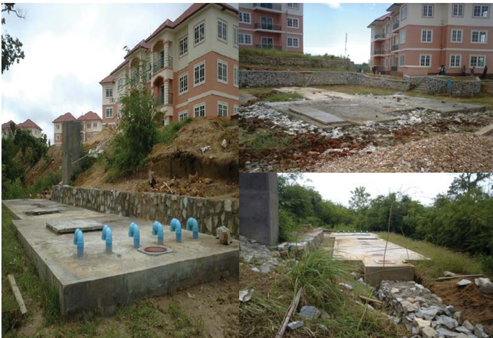
SEPTIC TANK IN NAYPYITAW
