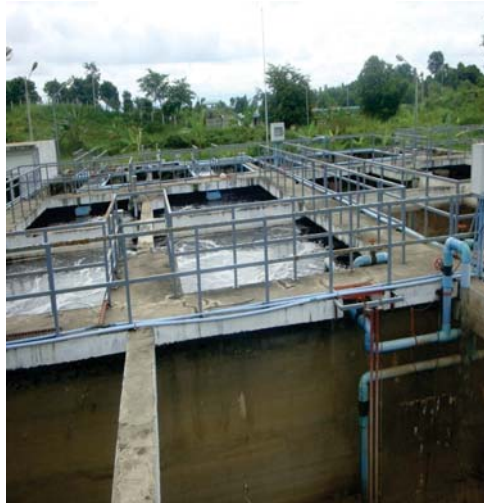
AERATION TANK OF SEWAGE TREATMENT PLANT
