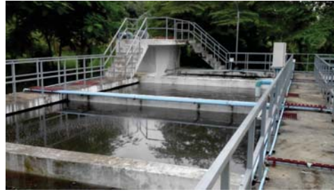
EQUALIZATION TANK FOR SEWAGE COLLECTION
