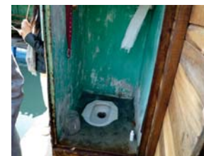
Toilet (Floating House) Vietnam
