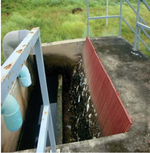
GRIT CHAMBER (INLET OF SEWAGE TREATMENT PLANT)
