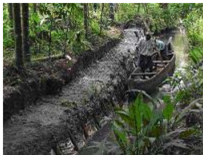
Bank protection work with “Neerkoova”
