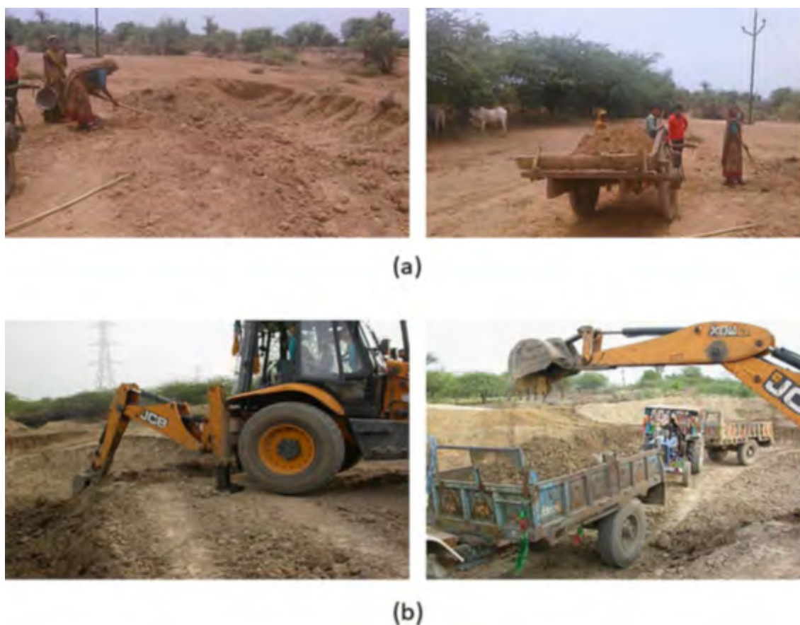
Figure 3. Desilting methods used for check dams before the 2015 and 2016 monsoons: (a) manual desilting of Badgaon check dam before 2015 monsoon, (b) mechanical desilting of Hinta check dam 2016. © Yogita Dashora
