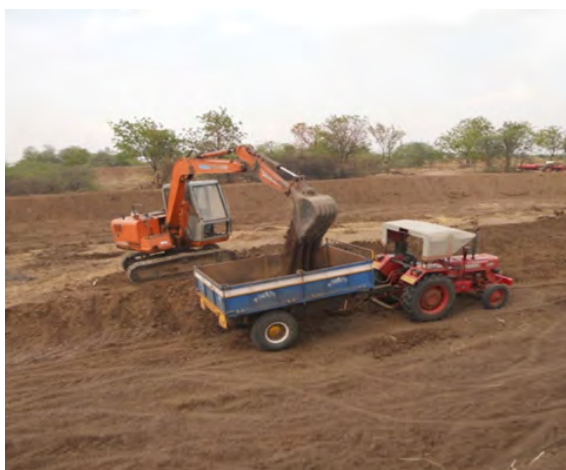
Removal of tank silt from check dam in Jalgaon K.P. NICRA village.
