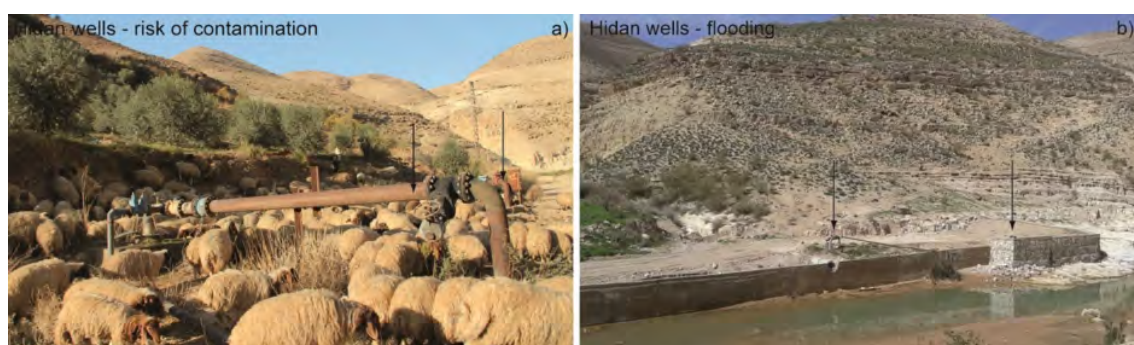
Figure 5. a) poor protected well in the Hidan wellfield surrounded by a sheep herd. b) flooded Hidan wellfield after heavy rainfall. © Julian Xanke
