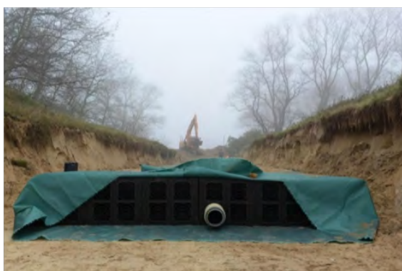
Figure 4 (a) Construction of 'subterranean infiltration' in water catchment of St-André (Koksijde). © IWVA
