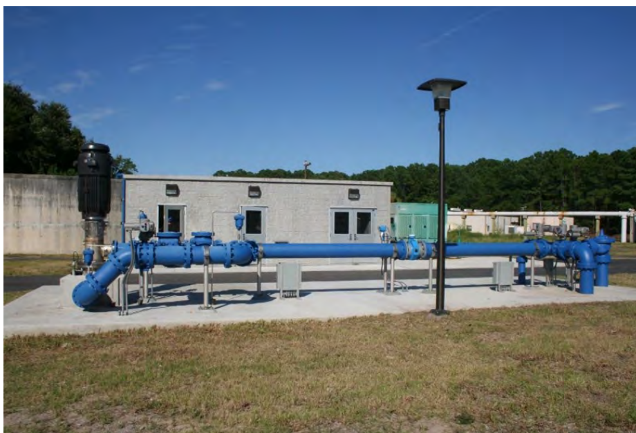
Figure 1. Well ASR-1 at Royal James, with pump, motor, wellhead piping, equipment shelter for electrical and SCADA controls, disinfection and emergency engine. © David Pyne
