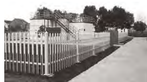
Decentralised wastewater treatment facility in Jiaxing City, Zhejiang Province
