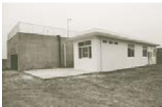
Domestic wastewater treatment facility constructed in Deyang city of Sichuan Province
