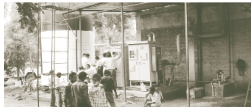
Installing heat pump in India
