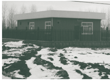
Waste water treatment facility in Weihai city
