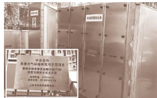
Model facility for oil smoke and odour treatment set up in Shanghai Academy of Environmental Sciences
