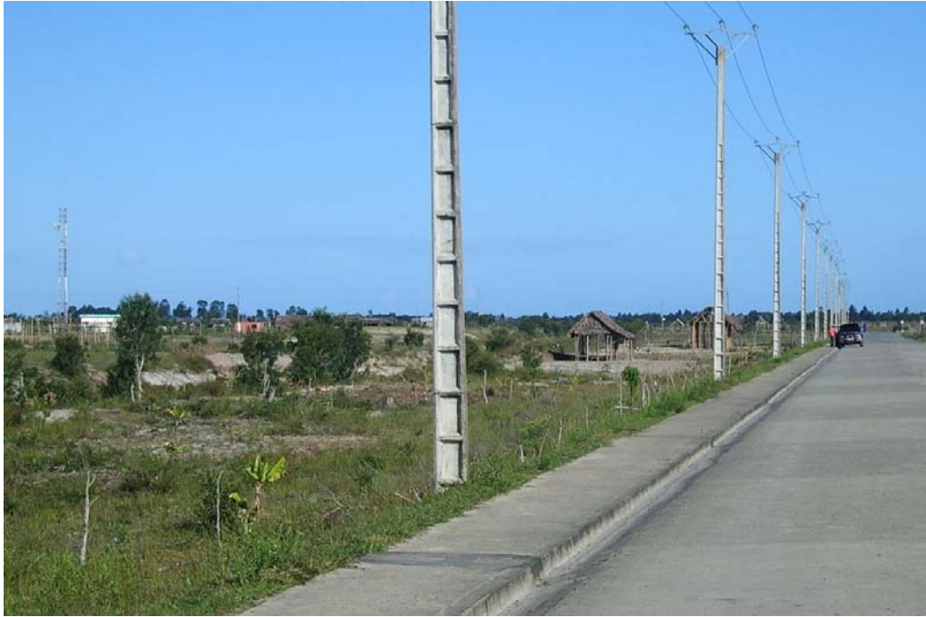
Plant Construction Site (planned)
